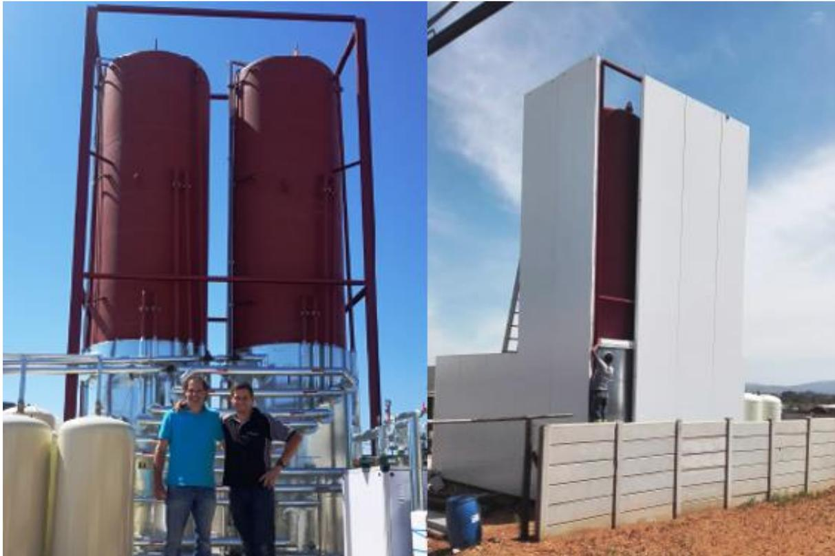
**Two locally manufactured 20 m<sup>3</sup> hot water storage tanks and a solar station were added to the solar field (left photo) put up at the tannery. Cellulose fibre, sourced from recycled newspapers, was then used to insulate the space between the housing and the tanks, reducing overnight heat loss to as little as 1 °C (right).**
