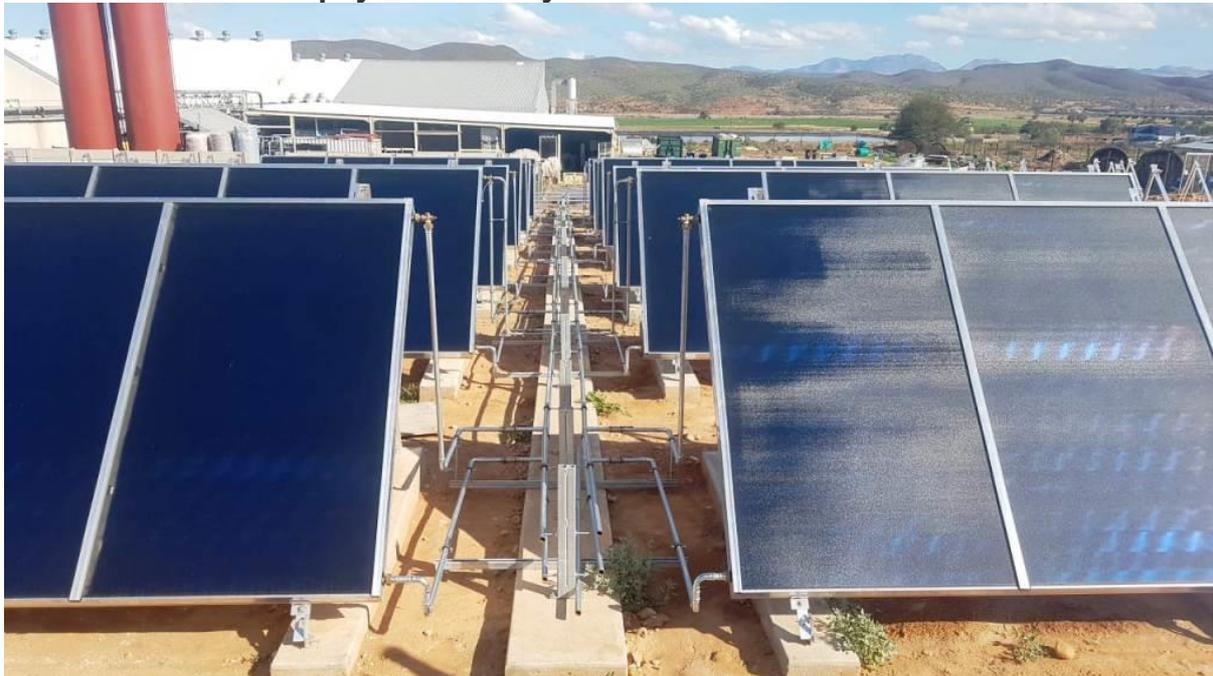
**The 600 m<sup>2</sup> of collectors installed at Klein Karoo meet 55 % of the tannery's heating needs. These ground-mounted units produce 10 % more than they would have if they had been installed on its factory roof.**
